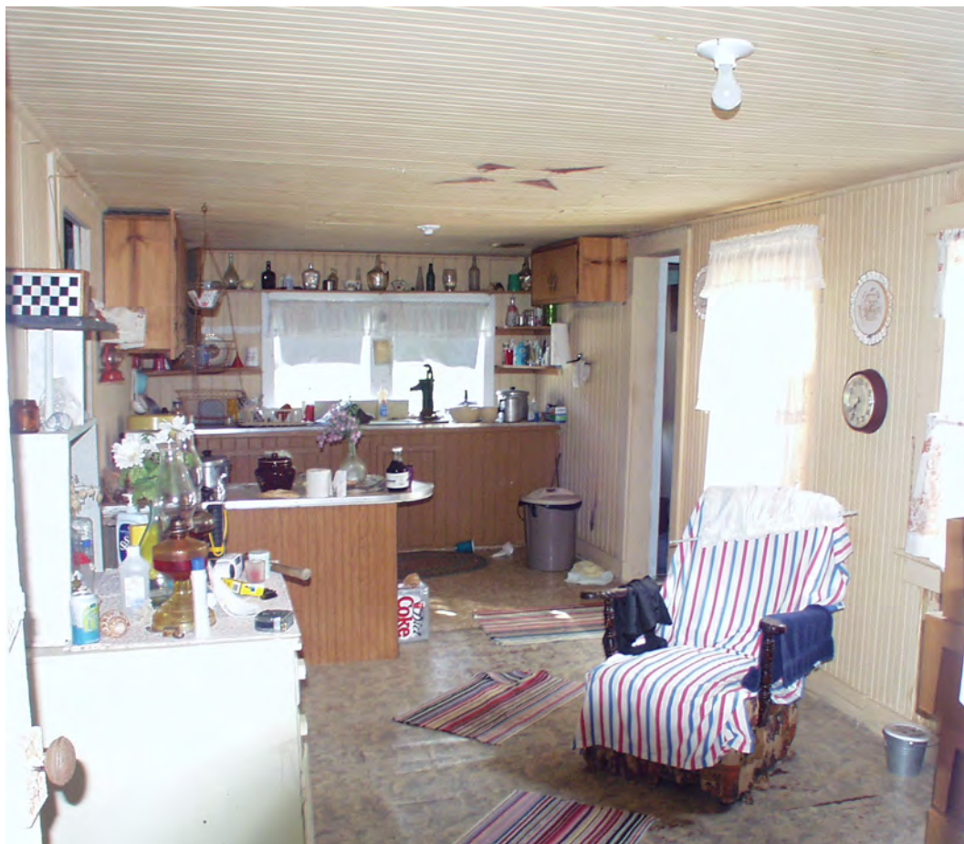
Figure 33 View to northwest in main room. (NPS-SERO-CRS, 2002)
