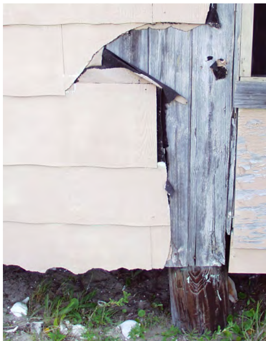
Figure 28 View of south corner of house showing original siding at center, asbestos siding at left, and modern plywood at right. (NPS-SERO-CRS, 2002)
