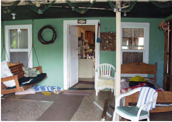
Figure 32 View of front porch. (NPS-SERO-CR, 2002)
