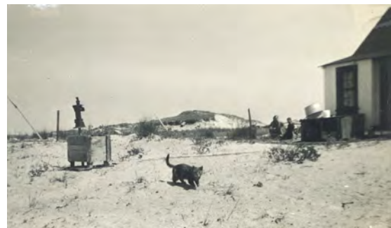
Figure 18 View at rear of O’Boyle House, 1941, showing bath at the end of the back porch. (CALO Coll., #30)
