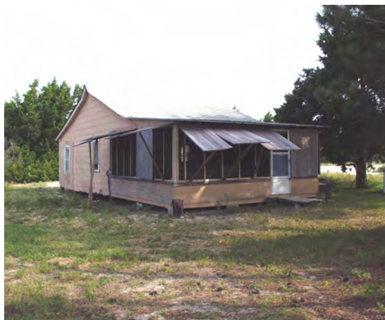
Figure 24 View to north of O'Boyle-Bryant House. (NPS-SERO-CRS, 2002)
