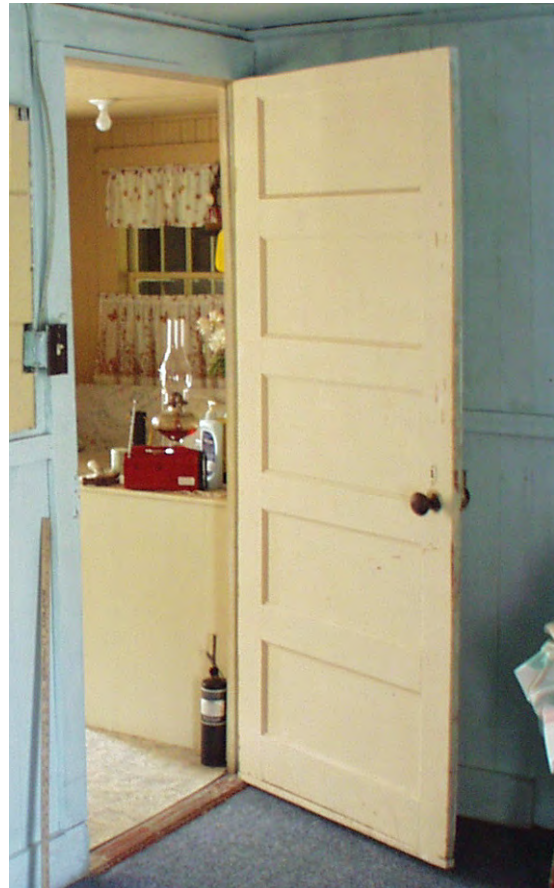
Figure 30 Five-panel door at Room 103. (NPS-SERO-CR, 2002)
