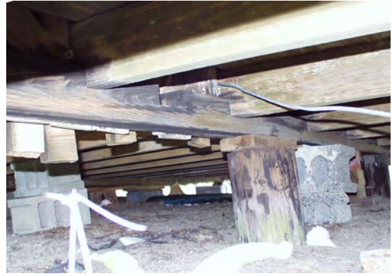
Figure 27 View of front sill of original house. Original siding extends below the bottom of the sill to left of center in this image. (NPS-SERO-CRS, 2002)
